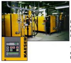
In the air center, seven KAESER screw compressors with state-of-the-art air treatment and control engineering are installed.
