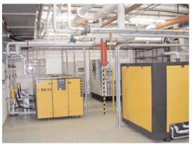
capacities of the machines. Three BS 51 screw compressors with a capacity of 5.3 m<sup>3</sup>/min each and a DS 141 SFC with 13.3 m<sup>3</sup>/min were installed. The DS
