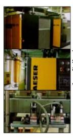
The compressed air center equipped with four KAESER screw compressors, booster and air treatment plant (upper and center).
